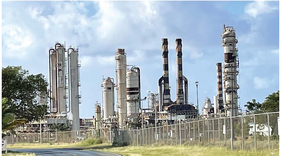
Figure 12: Closed Oil Refinery on U.S. Virgin Islands
